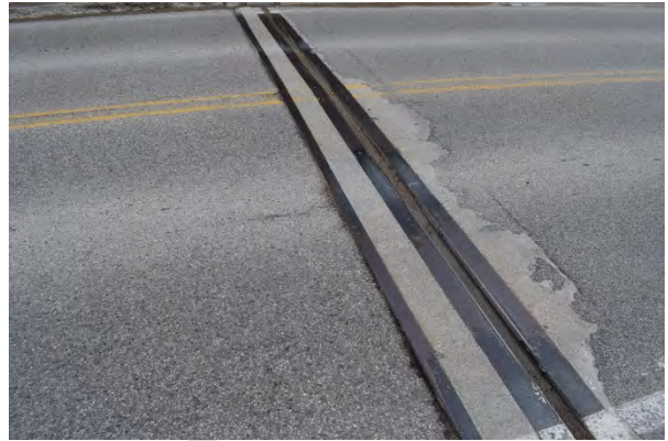
Plate 35: Expansion joint on west side of the bridge
