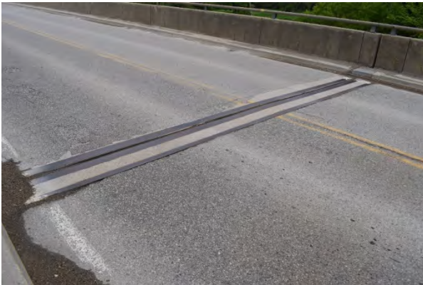
Plate 36: Expansion joint on east side of the bridge
