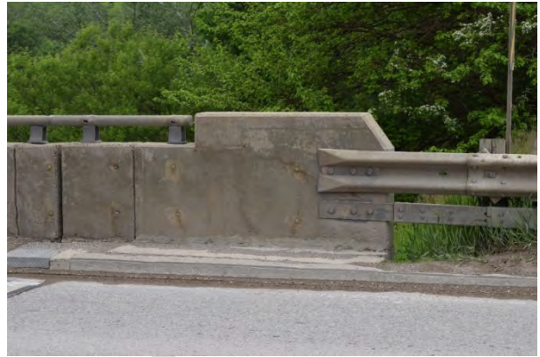
Plate 31: Steel guardrails attached to bridge parapet wall on northeast side of bridge
