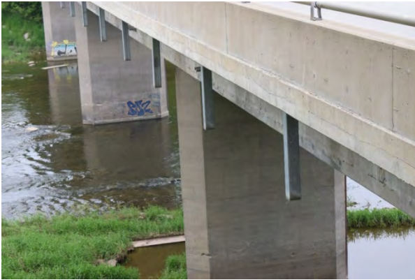
Plate 34: Metal deck drains along bridge
