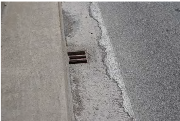
Plate 32: Top of metal deck drain
