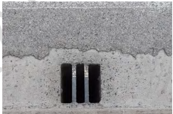
Plate 33: Detail of top of metal deck drain
