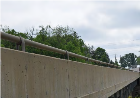
Plate 30: South concrete parapet wall and steel rails looking northeast
